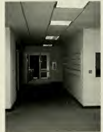
The original building was a squat rectangular structure with precast panel walls, few windows, and little daylight. Photograph: Bruce Gora
